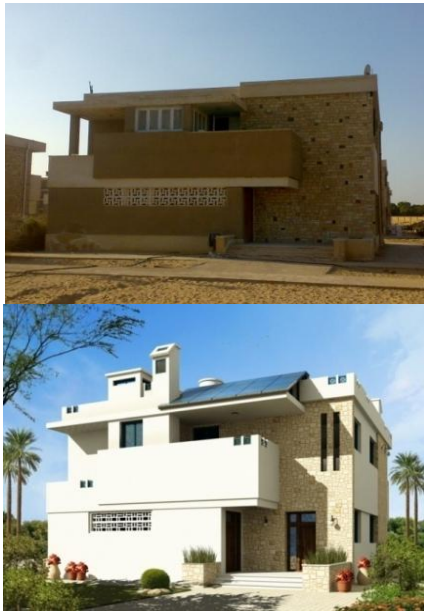
Fig. 13. Wardan staff housing unit perspective (before & after renovation) [9]
